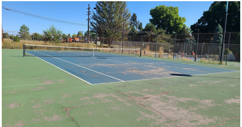
Existing Condition of Courts
